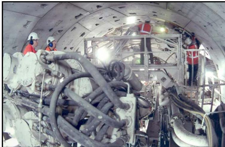
Following recent tunnelling experience in London, CLRL will utilise Earth Pressure Balance TBMs except for the Thames crossing where a Slurry machine will be employed
